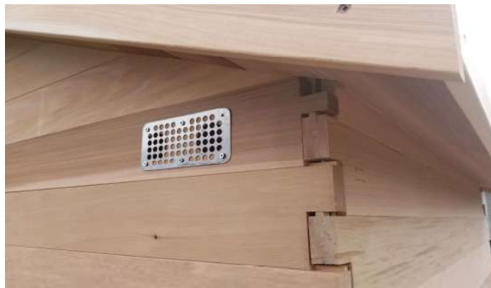
Install the other Stainless Vent cover over the outlet holes on the outside using 1-1/2" stainless steel screws. (6pcs)
