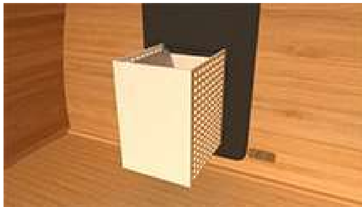
Inlet beside wood heater on Back wall
