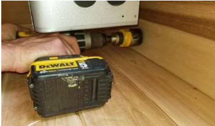
Drill inlet holes centered underneath the heater. (if sauna is being installed with a wood heater, drill close to the side of the heater)
