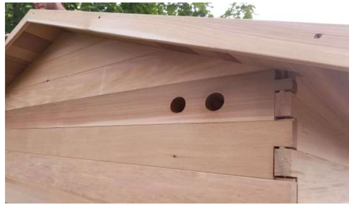
On the wall away from the heater, close to the top, drill the outlet holes in the same manner as the previous step
