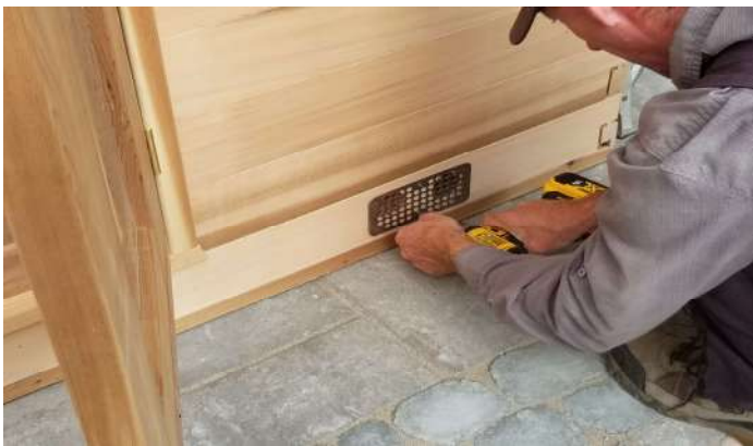
Install 1 of the stainless steel vent grills over the inlet holes on the outside of the sauna centered over the holes using 1 1/2" screws. (6pcs)
