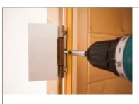
Before attaching the door, place it in the opening and insure that there is a 1/8" gap between the glass and the door header, and about a  $\frac{1}{2}"$  gap at the floor. With one person holding the door up (or set on  $\frac{1}{2}"$  spacers at the floor) screw the hinges into the vertical hinge post using the screws included with the hinges. Secure one screw in each hinge and then close the door to be sure of the fit. Once the fit is verified secure the remaining screws.
