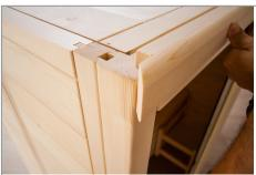
Find 4 pieces of roof trim. Place the long piece with the two 45° angles on the front, and the two short pieces on the sides. Attach to the sauna using 3.5x40 screws, (4) in each long piece and (2) in each short piece. Screw from the top and into the roof sections. NOTE: The rear piece of trim is generally not used as the sauna is placed against a wall. However, if you use the rear trim then it will need to be cut to fit around the two side pieces of trim.
