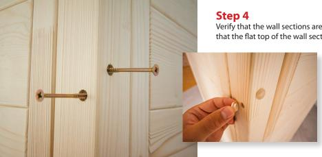
Verify that the wall sections are square to the rails, perpendicular to each other, and that the flat top of the wall sections and corner posts align. Using a cordless drill
