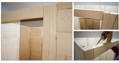
Find the glass window section and position into the groove of the vertical wall section post. Then, position the header for the door so that the groove goes over the top portion of the glass window. Insure that the top of the header is flush with the tops of the wall sections and screw into place using 4x70 screws inserted on an angle.
