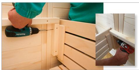
Find the vertical bench section and position in front of the vertical bench supports. Using (4) 4x60s screws, from the backside attach the vertical bench section to the vertical bench supports as shown.
