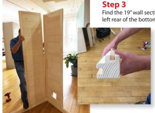
Find the 19" wall section with the square cut out hole and position on the left rear of the bottom rail. NOTE: These instructions place the door on
