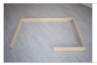
Locate the (4) bottom rails and position as shown. Overlap the corner joints and be sure the rails are square to each other.
