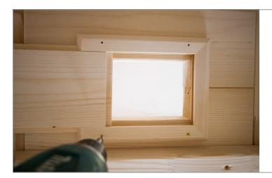
Locate the vent cover and position over the wall opening. Attach with (4) 3.5x40 screws.
