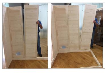
Place two additional 19" wall sections on the back wall of the sauna. There will be no screws used in these sections, but be sure the wall sections are placed firmly to the bottom rail so that the flat top sections are flush with each other. NOTE: In step 14 you will begin to secure the wall sections together using the roof support rails.
