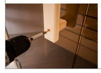
**Step 29**Install the handle on the door using the screws provided.
