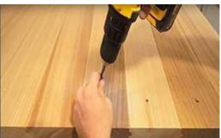
Secure the roof staves into the front and back walls using 2 ½" (64mm) screws.
