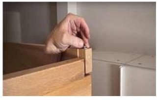
Place the washer then the nut on the threaded rods and tighten with the wrench. Do not overtighten!
