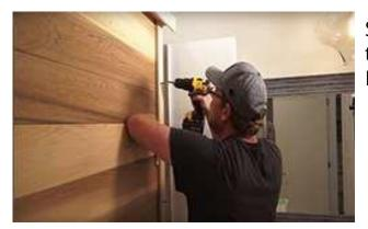
Secure the outer trim pieces to the outside corners of the sauna using  $1 \frac{1}{2}$ " (38mm) screws. Repeat for all 4 corners.
