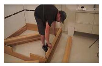
Once the front and back staves are installed, insert another side wall stave on either side. Repeat this process (Front, Back, Sides) until you reach the fourth row on the front of the sauna.
