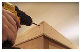
Line the front roof trim with the side trim ensuring they are flush and secure with 1  $\frac{1}{2}$ " (38mm) screws. Repeat for the back roof trim.
