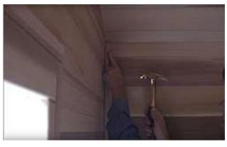
Measure each of the 4 corners inside the sauna and cut the interior trim pieces accordingly. Fasten the interior trim pieces with the provided finishing nails.
