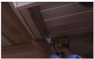
Repeat the process if adding an L shaped bench. Secure the L bench to the back wall bench from underneath with 2 ½" (64mm) screws.
