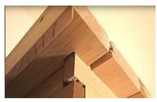
When you reach the opposite side of the roof, tap the remaining roof trim piece flush into position using the rubber mallet.
