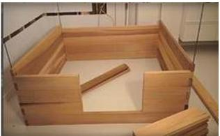
When you get to the 4<sup>th</sup> row on the front wall, it is time to install the door. Ensure the sauna is square as you assemble the walls to make future steps easier.
