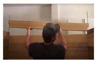
The staves should get easier to install and the sauna much more stable as you progress upwards.
