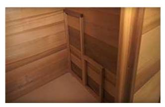
Bring in the bench brackets. Fasten the bracket to the back wall using 2 ½" (64mm) screws in the pre-drilled holes ensuring the bracket is snug to the back wall.
