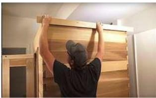
Place the roof trim on top of the side wall. The holes will go over the threaded rods.
