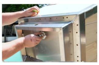
Thread the short piece of pipe into the drain hole from the bottom of the cold plunge tub.
