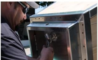
Screw the 90° elbow onto the short pipe.
