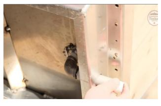
Thread the long piece of pipe into the elbow.
