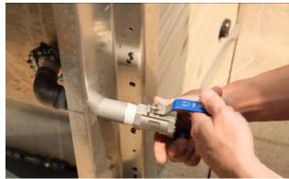
Screw the valve onto the end of the long pipe.
