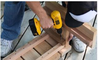
Ensure the stair support is flush at the back of the step and secure with  $2 - 2 \frac{1}{2}$ " (64mm) screws.
