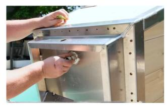
Thread the short piece of pipe into the drain hole from the bottom of the cold plunge tub.
