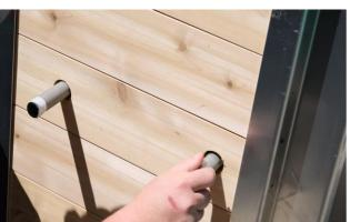
Wrap 3 layers of thread tape around both ends of the threads on the 2 remaining long pipes and thread them into the holes on the side of the tub.
