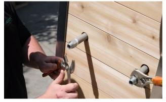
Thread a quick connect onto each of the long pipes.
