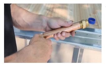
Wrap 3 layers of thread tape around the threads on both ends of the long pipe.
