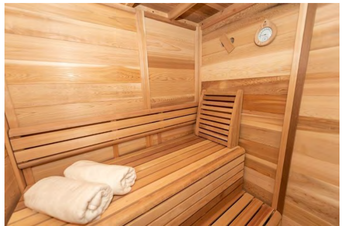
Outlet vent high on opposite wall of heater.
