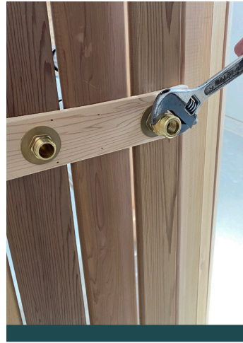
15. Twist on the adaptor fittings on both inlets and tighten with adjustable wrench.
