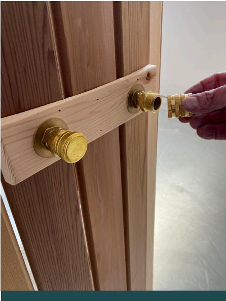
17. Twist swivel connector onto the other adaptor and hand-tighten. Attach a garden hose to the swivel connector. Your shower is now ready to use.
